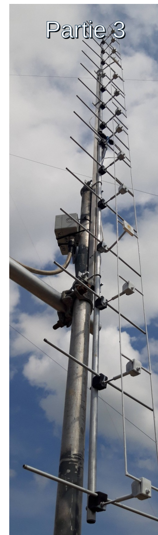
2x6 Quadlong 432 MHz gain 16dBi Az.71° El.11.4°
