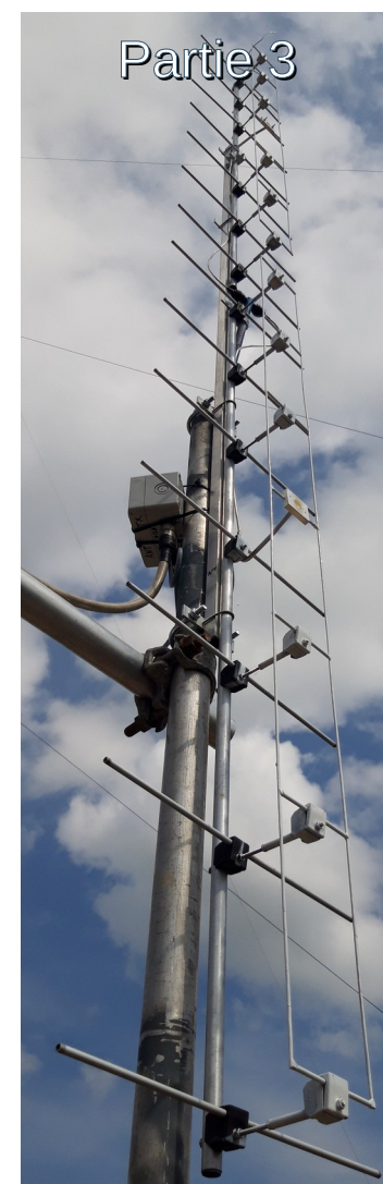
2x6 Quadlong 432 MHz gain 16dBi Az.71° El.11.4°
